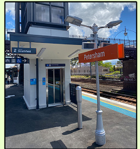
Petersham Station now has lifts from the platform to street level
