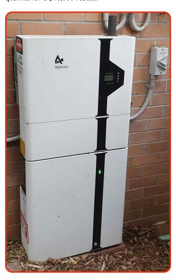
A 20kW battery is twice the size we need based on our current usage however, there are other considerations. You only get one bite of the cherry for the federal rebate and it runs out in 5 years. We have recently gone all-electric, disconnecting our gas and purchasing a heat-pump hot water system and induction cooker. We also have ducted air conditioning, so I wanted to build in some redundancy. The payback time for our battery is estimated to be 4.7 years.
